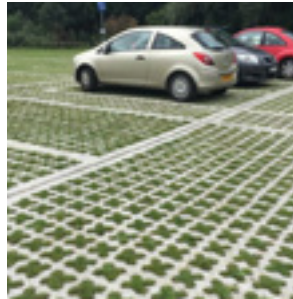
Use of Grass Crete paving to soften large extents of hard surface.
